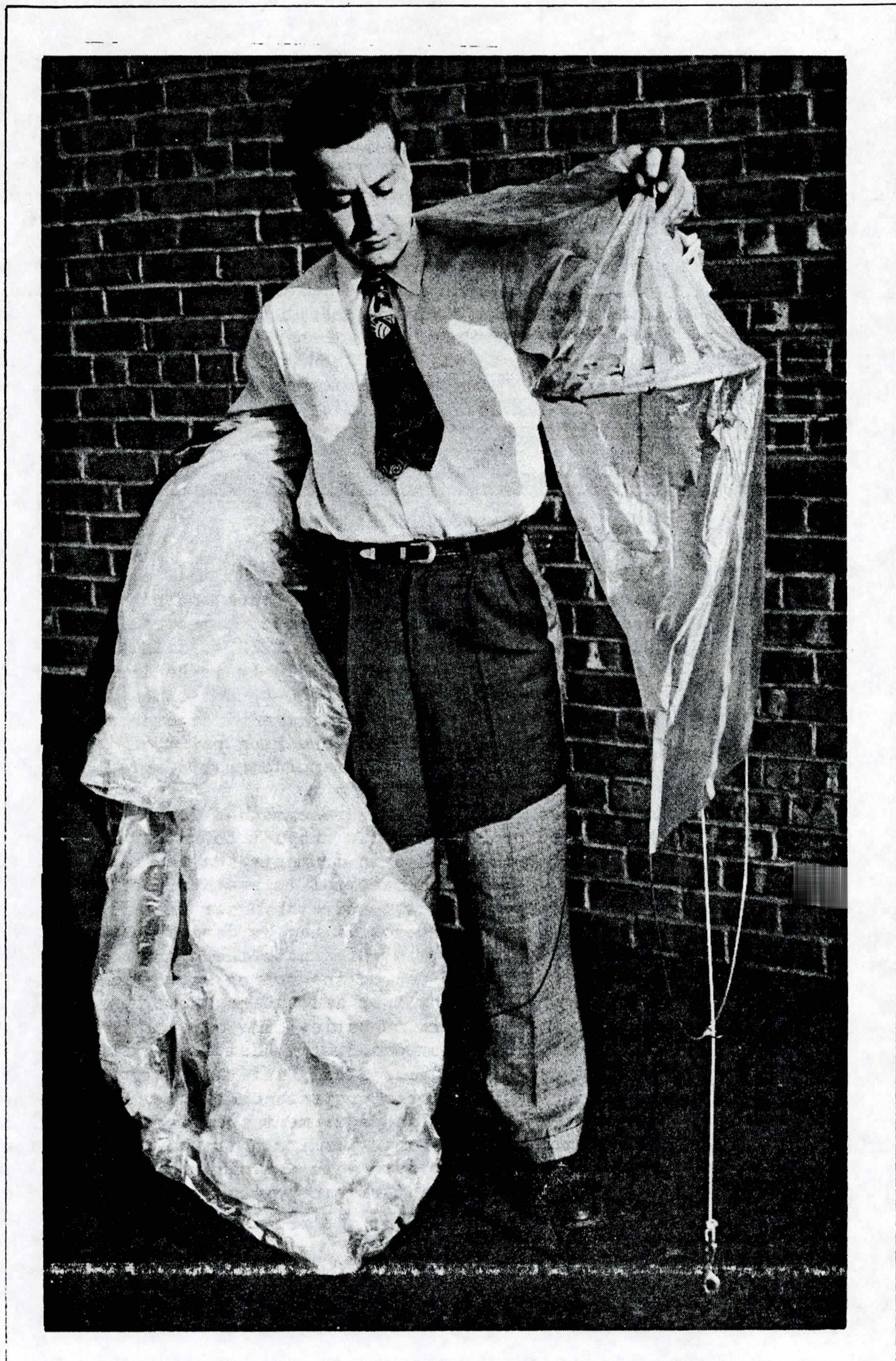
Figure 4 Two foot appendix, showing metal spring bow in position.
